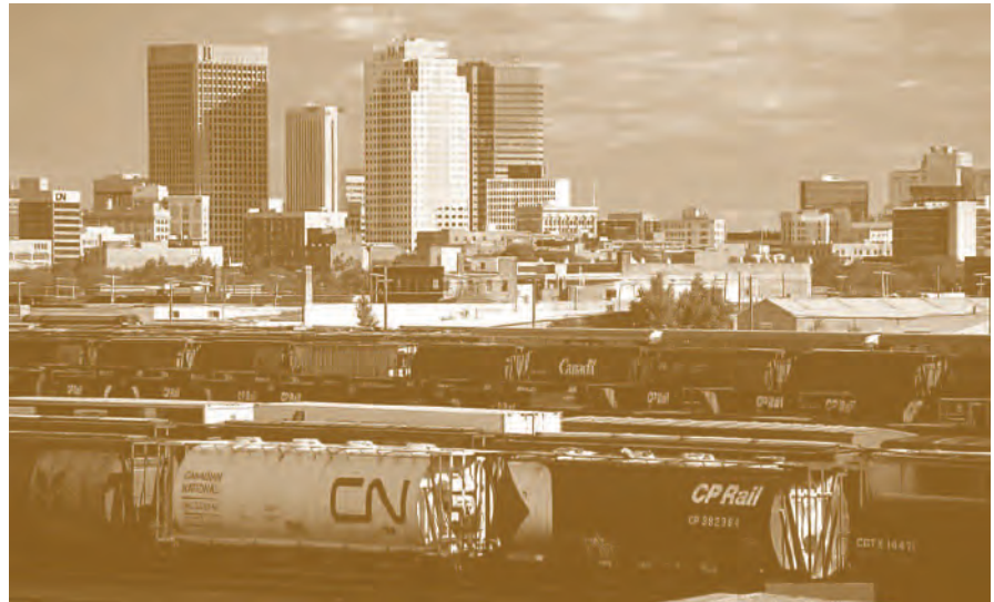
Centreport Canada will be a 20,000 acre inland port next to Winnipeg's international airport.
